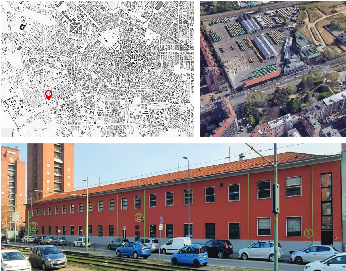
Figure 1. Location and site of the 'deposito ATM', Via Giambellino 121, Milan (Italy). Giambellino area within the city; location of the bus station and previous appearance of the building before installing the living wall, where section 1 and 3 will subsequently be covered by green wall and section 2 covered with an informative panel (credit: Paolo Pignataro).
